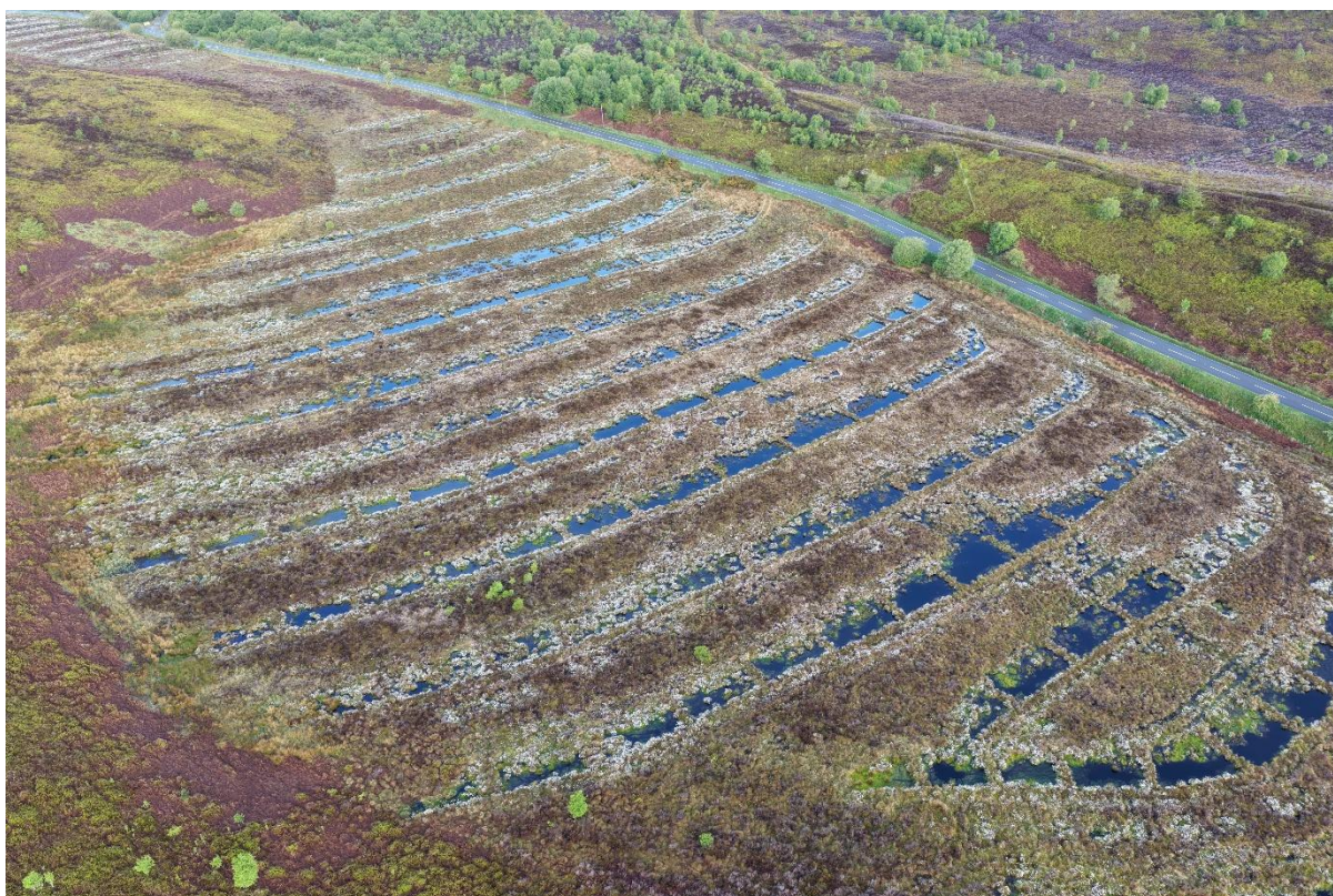
Figure 5. Contour Bunding at Llandegla Moor SSSI
